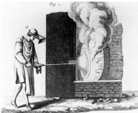
Figure 19.24. Before 1800, plate glass was made by spinning a glob of hot glass on the end of a rod, allowing centrifugal force to form a disc about 1.2 m in diameter. Panes were cut from the disc. Courtesy of Broadfield House Glass Museum, Kingsford, UK.
