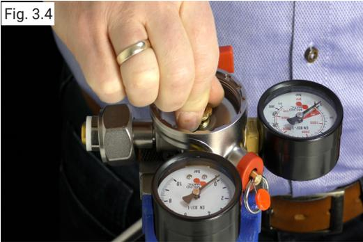
Fit the new Cartridge by turning it clockwise by hand.
