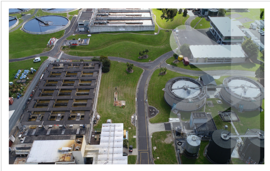
[그림 4-1] Pukete Wastewater Treatment Plant
