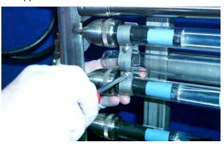
**13.** Place rubber washer on replacement UV Sensor. Insert replacement UV Sensor into sleeve, making sure all sealing surfaces are clean and undamaged.
