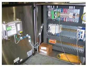
The PLC is programmed to provide safe and efficient control of the UV system's banks of lamps as it interfaces with the Power Distribution Center (PDC), Communication Control Boards (CCB), effluent flow signal, On-line UV Transmittance Controller and Sensor and Hydraulic System Center (HSC). Information from these sources is used to control the automatic dose-pace strategy for the UV lamp banks.
